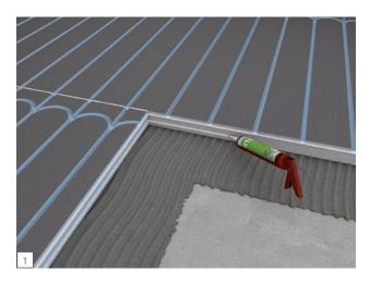
The wedi PreLine is laid across the full surface with a thin-bed mortar (recommendation: wedi 320 universal tile adhesive) and aligned. In wet areas, the building board joints must be fully and thoroughly bonded and sealed with wedi 610 adhesive sealant (recommendation: one bead of wedi 610 underneath the milling groove and one bead level with the milling groove).
