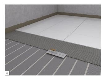
Ceramic tiles with a minimum size of  $10 \times 10$  cm can be laid on this surface. The wedi PreLine can be tiled directly after reinforcement without further pretreatment. Laminate or complete parquet must be laid as a floating floor.
