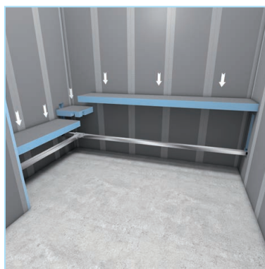
Use wedi 610 to seal/bond all elements to profiles, to each other and to the walls.
